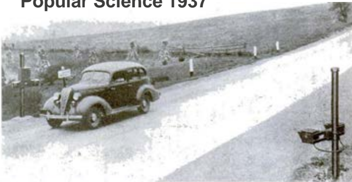
Passing vehicles intercept parallel beams of light and are counted by a photo-electric recording device
